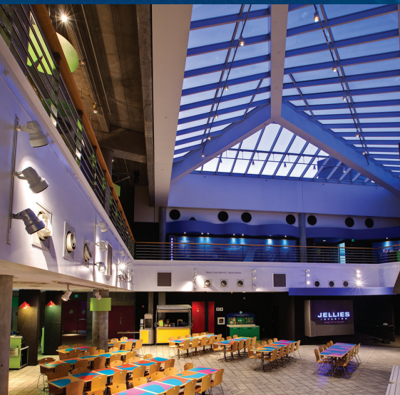
Longer-lasting and more efficient LED lighting in the café atrium means fewer bulb replacements and lower maintenance costs.
